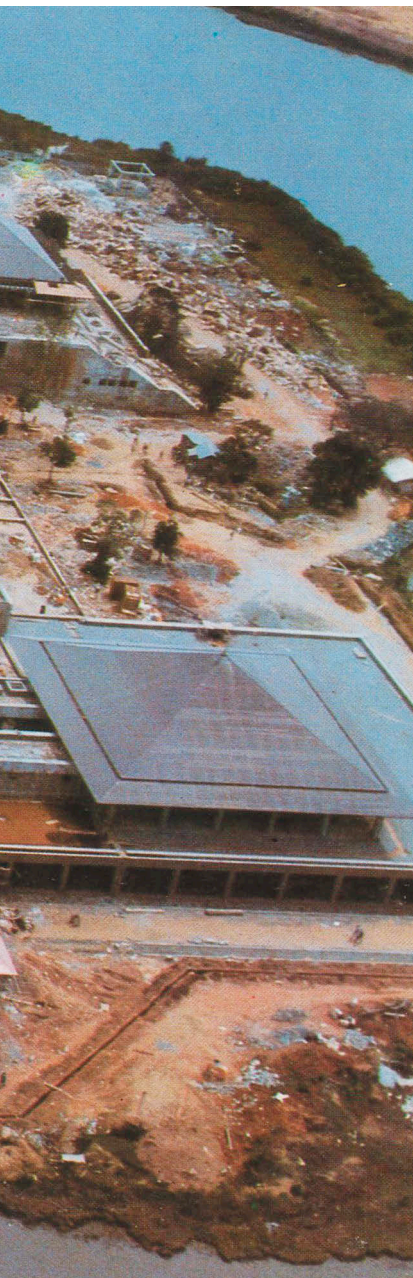
An aerial view of the Parliament building under construction.
